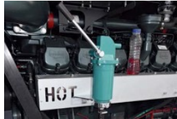
Ölabsaugpumpe Oil drain pump
