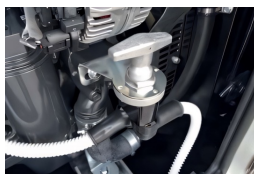
Batterieschalter Battery isolator switch
